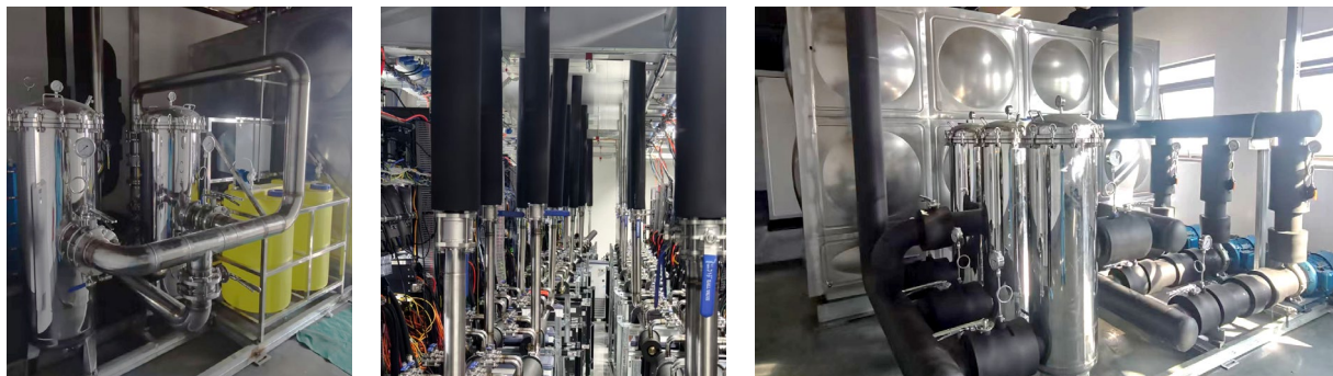
Closed-loop Cooling Water System Energy-saving Retrofit Project
